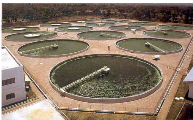
Figure 5: A standard design for industrial production of spirulina
